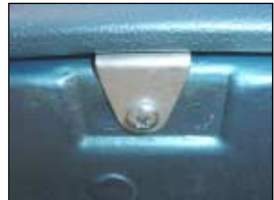
Installed panel clip
